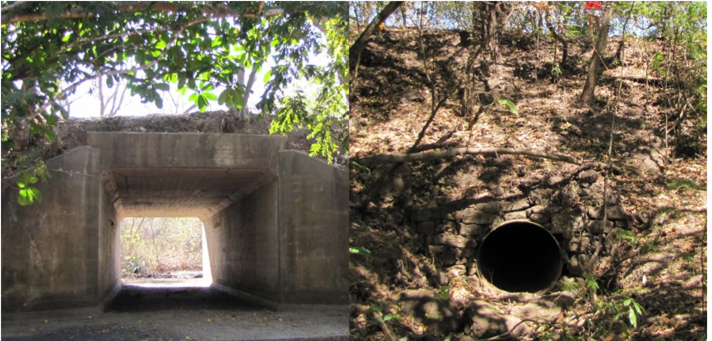
Figure 2. Culverts or drainage structures built on the 30-kilometer segment of the North Inter-American Highway. These structures are built according to the rivers and streams running across roads, rather than to animals that may cross the road.
